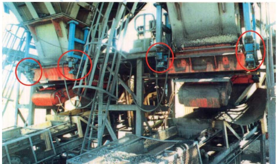
*Discharge chutes on coal silos in New South Wales, hanging on AB 50 mounts*
