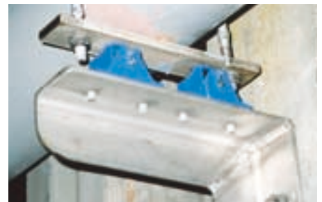
Elastic suspension of hot steam pipes on anti-vibration mountings type V-38 (compensation of heat-induced expansion).
