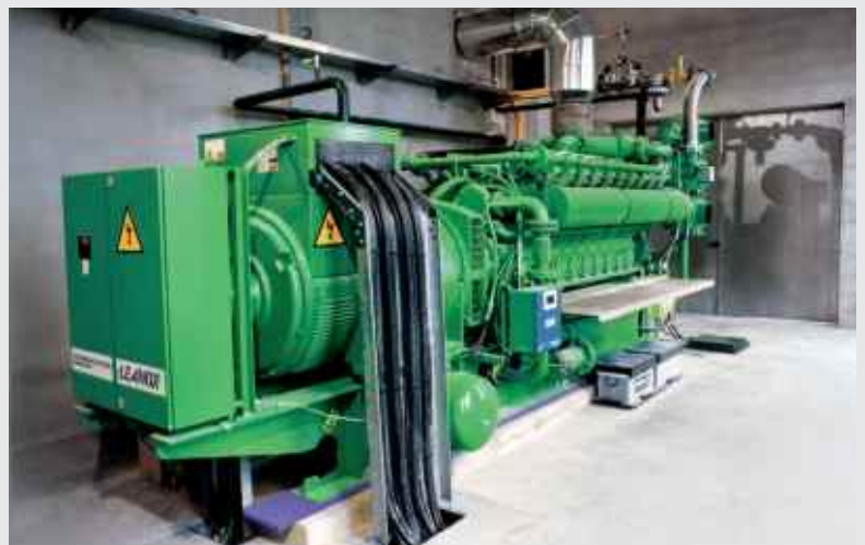
Machine foundation bearings
