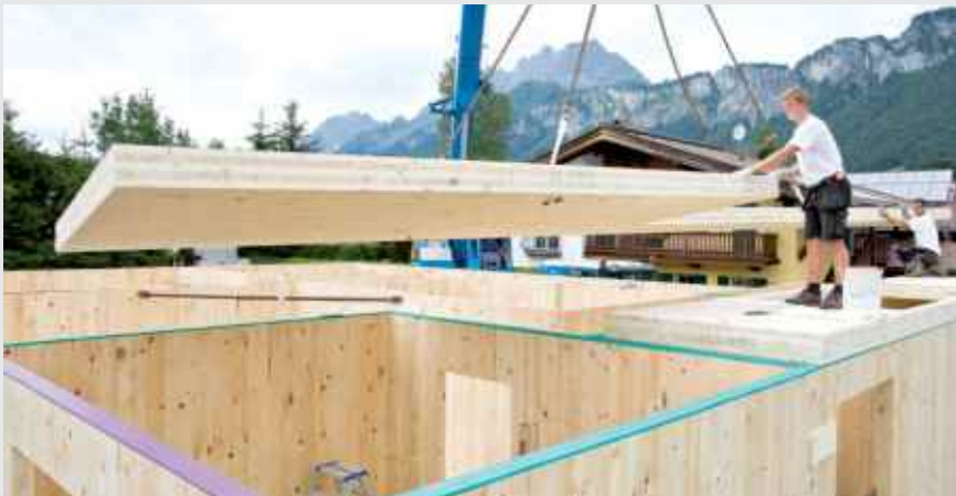
Sylodyn® strips for decoupling of the flanking transmission
